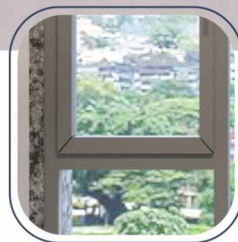
45°Degree Corner Joint
